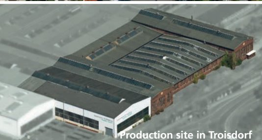
Production site in Troisdorf
