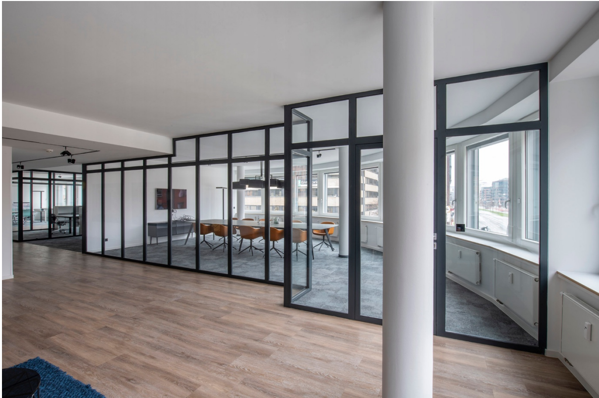
The stable and transparent WP 50 cold steel door and partition system (Pictures: Peter Kanthak)
